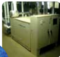
75kW Cogeneration System
