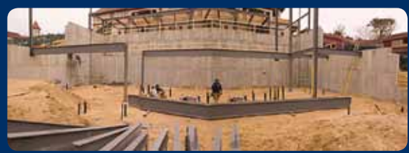
Foundation for the Ocean Edge Conference Center
